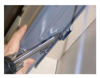
Remove wand. If the blind has a wand with a connector clip, use needle nose pliers to grasp the wand connector clip below the tilter stem. Twist the clip to disengage from the grooves in the tilter stem.
